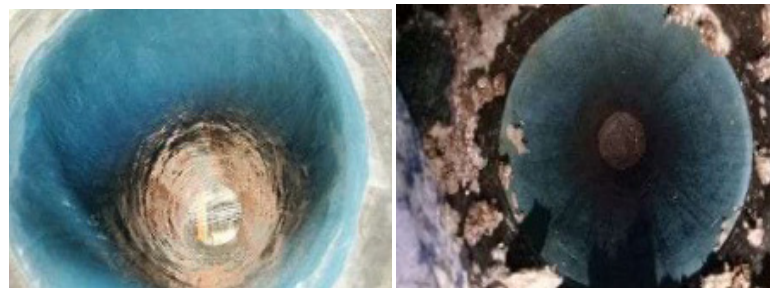
Figure 15. New coating, Chesterton combination of ARC S1HB and after six months of use, the coating is still in good condition.
