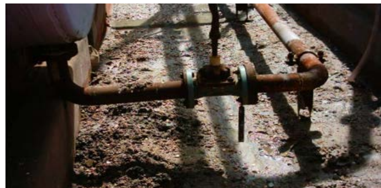
Fig 2.6 Acid attack of concrete in sulfuric acid containment
