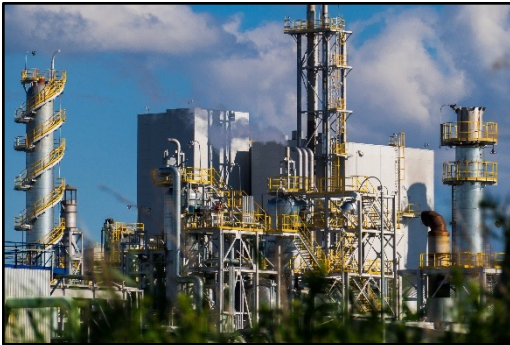
The pump seal failure occurred nearly every month.
