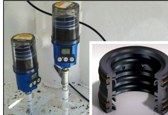
Chesterton Lubri-Cup™ EM and 615 HTG installed.
