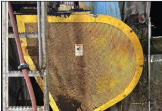
Front view of stuffing box with safety guard during operation.
