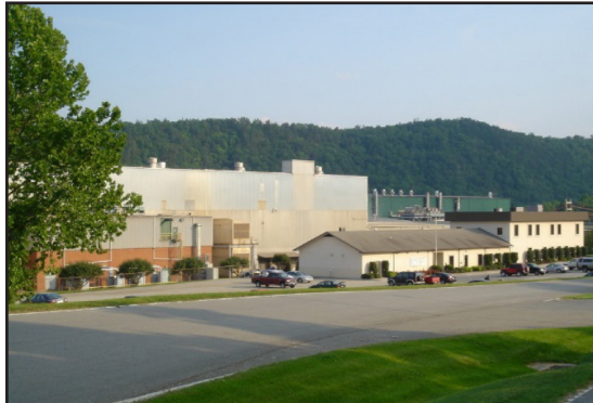
Paper mill was challenged with unreliable sealing with the agitator.
