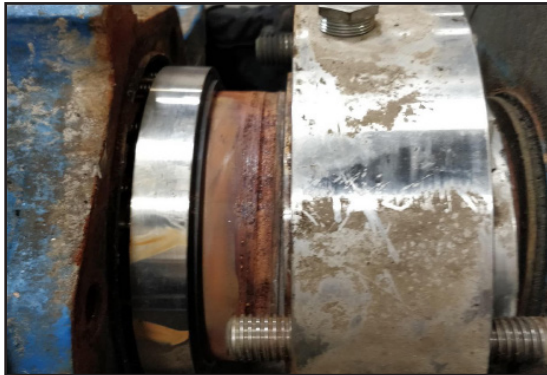
Split case pump with solid mechanical seal.
