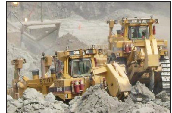
Caterpillar® D11R equipment performing leak free in operation.
