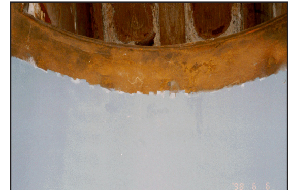
Second coat of ARC S7 applied, completing the project
