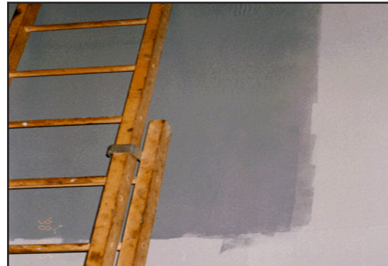
First coat of ARC S7
